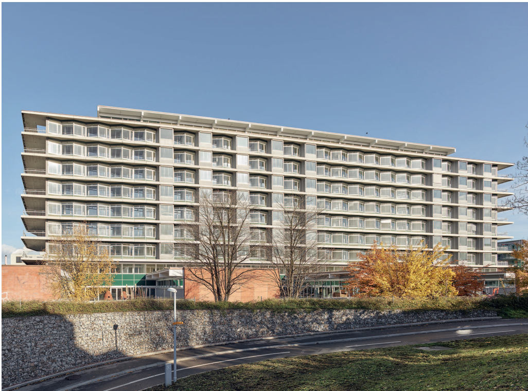
Fig. 1 Aussenansicht Südfassade. Exterior view of the south façade. (© Ariel Huber)
