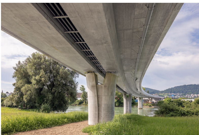
Fig. 5 Neue Reussbrücke, Blick von Norden Richtung Reuss. New Reuss bridge, view from the north towards the Reuss.
