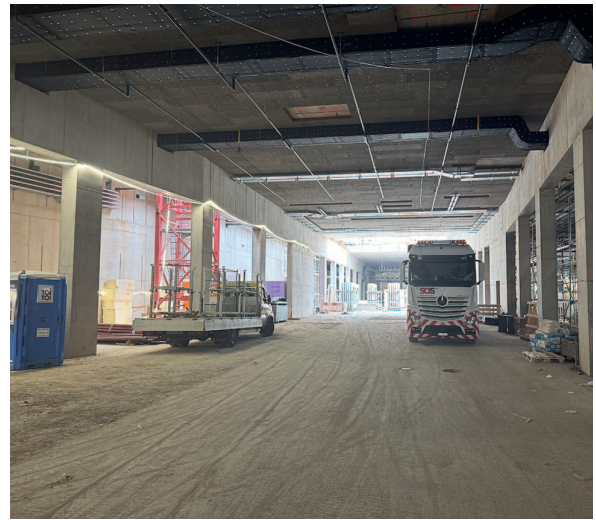
Fig. 7 Die 145 m lange Depothalle diente während des Baus dem Materialumschlag. The 145 m long depot hall was used for material handling during construction.
