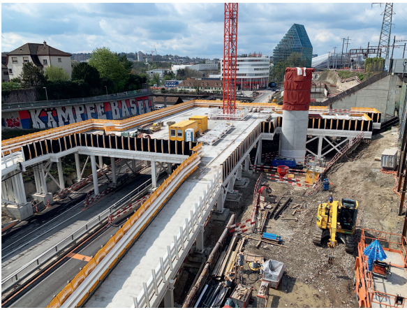
Fig. 5 Installationsplattform. Working platform.
