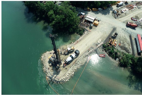
Fig. 6 Erstellung Pfeilerfundation mittels Ford. Construction of pier foundations using a ford.
