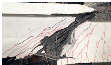
Shear failure in the beam web.
