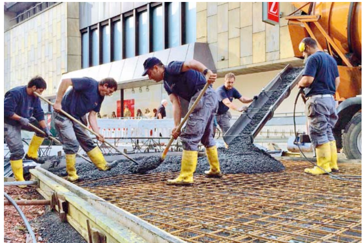
Abb. 9: Betonage
