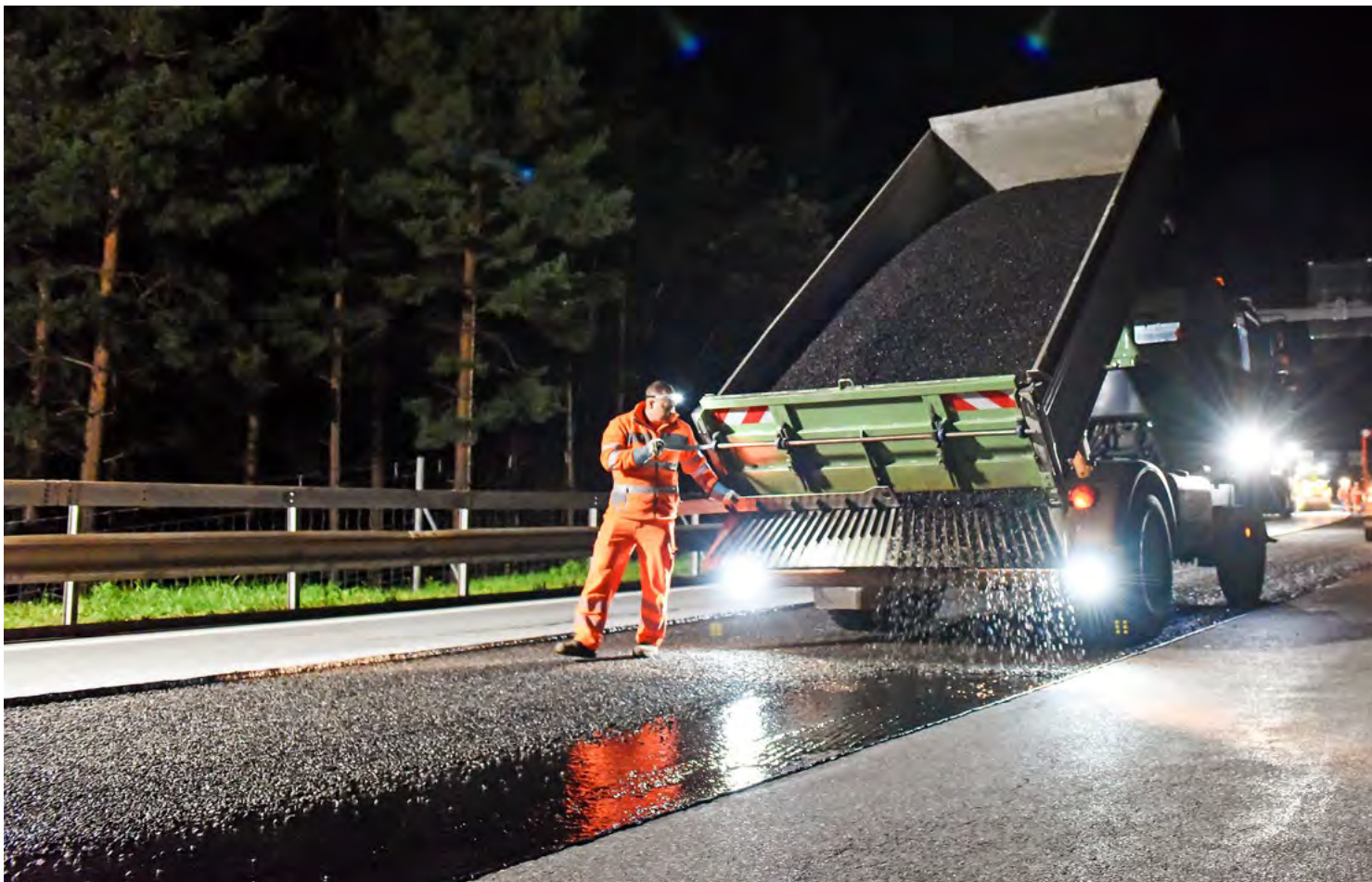
Applikation der SAMI (Stress Absorbing Membrane Interlayer)
